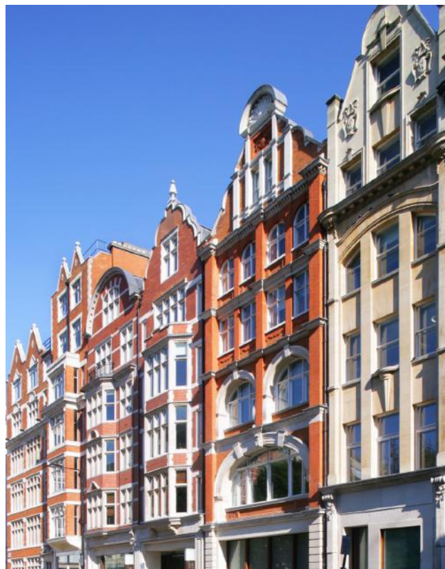
Photo of 4 th floor (rear) yet indicative of 2 nd & 3 rd floors after refurbishment (unless fitted space desired)
